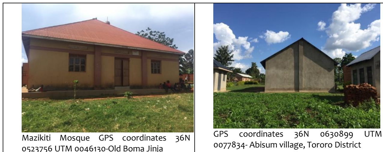
Figure 9.2: existing shrines and houses
